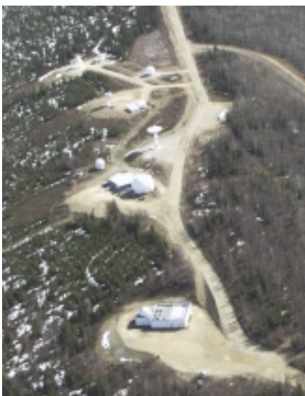
The Alaska Ground Station (AGS) located at the Poker Flat Research Range (PFRR) near Fairbanks. (Source: Univ. of Alaska)
