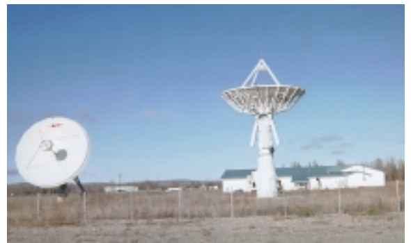
Space Imaging's ground station located south-east of Fairbanks with the tracking antenna used to communicate with the polar-orbiting remote sensing satellites in the background and the antenna that is directed towards a communications satellite in geo-synchronous orbit in the foreground. (Source: Space Imaging)
