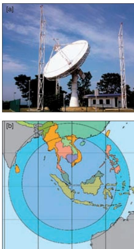
**Fig. 9 (a)** - The large 13 m diameter X-band antenna of the CRISP ground receiving station located in Singapore. (Source: CRISP)
